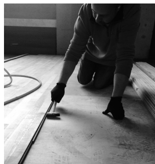
Attaching the spline
